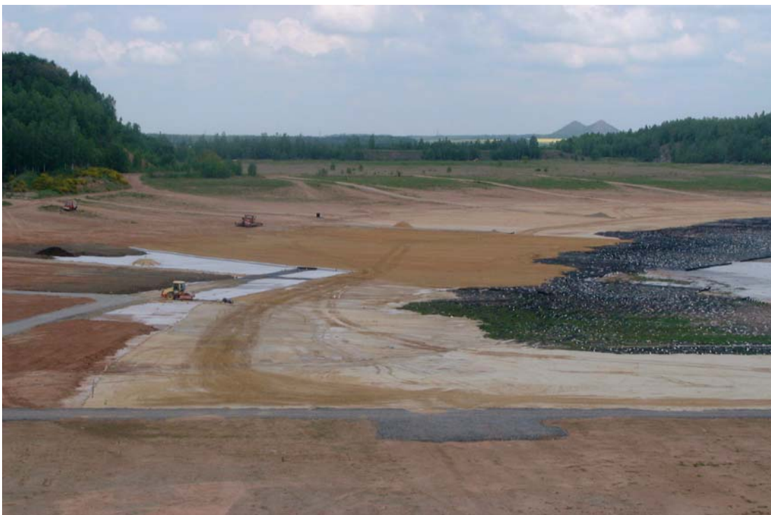
Picture 7: Wismut site under remediation, Germany.
