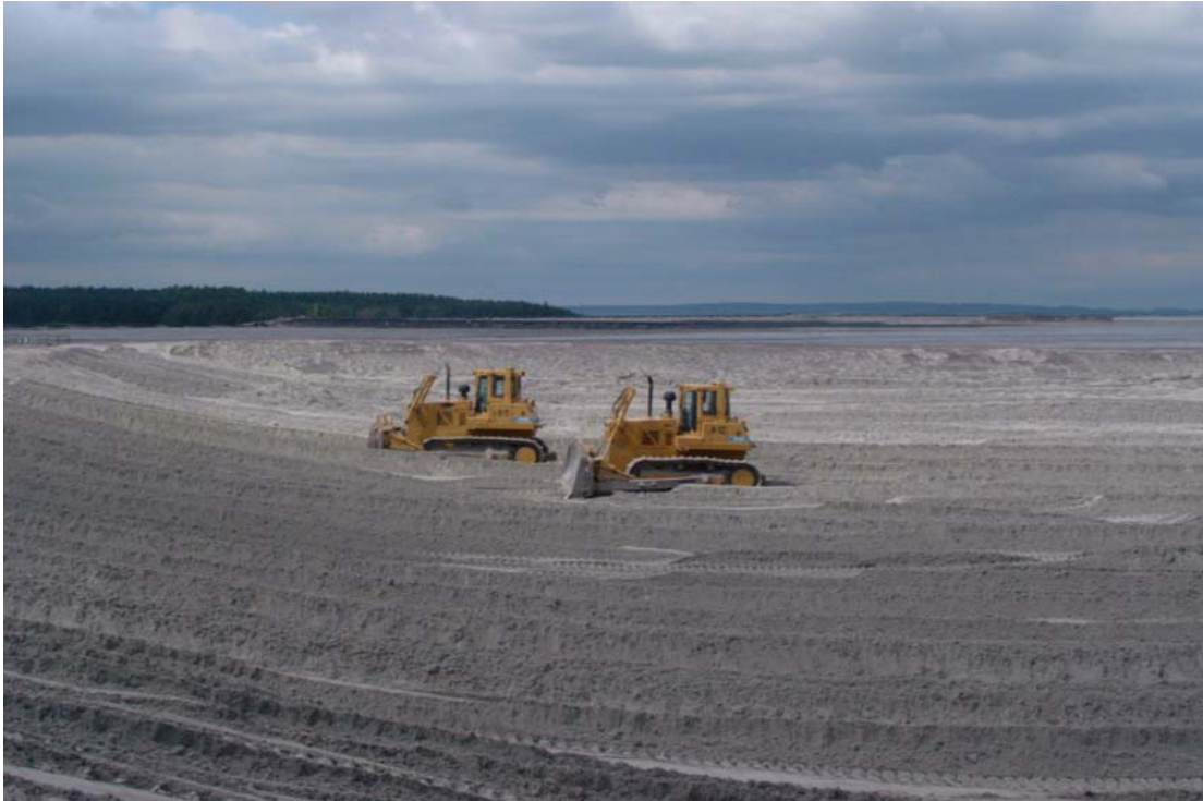
Picture 6: Increasing the height of the tailings dam in Żelazny Most, Poland.
