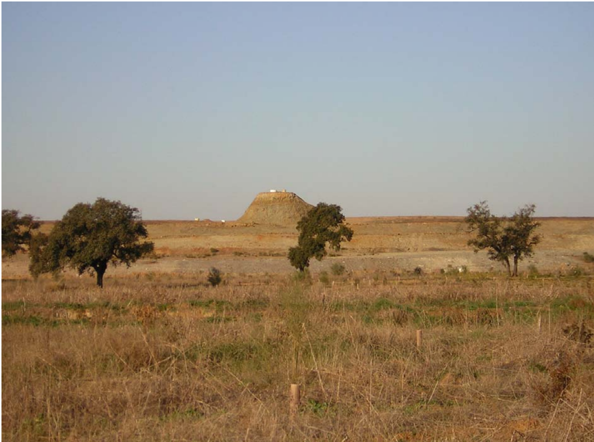
Picture 4: The remains of the tailings dam embankment in Aznalcóllar, Spain.
