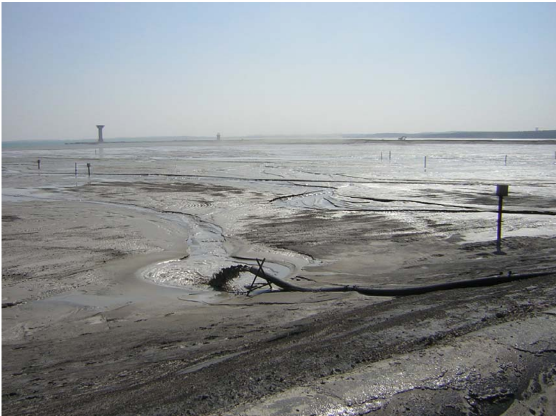
Picture 5: Spigotting outlet in Żelazny Most, Poland.
