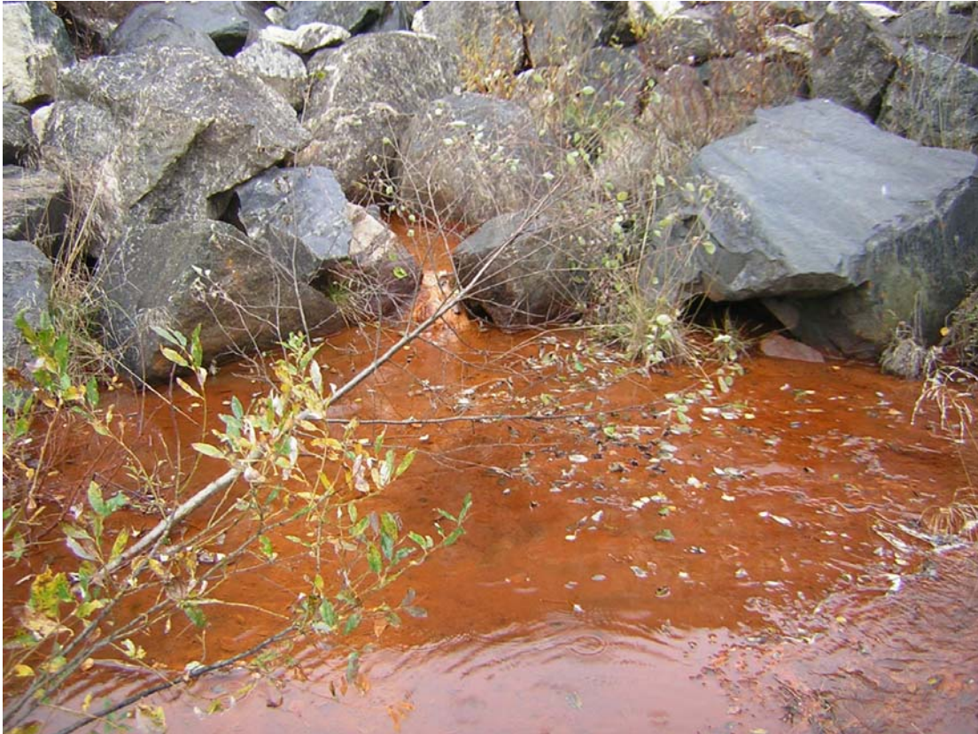
Picture 8: Seepage in Siilinjärvi TMF, Finland.
